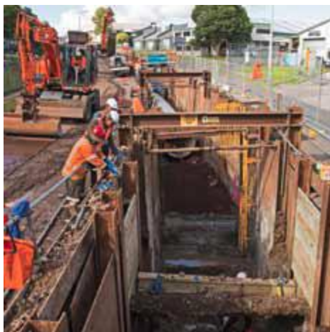
The NEC-procured first stage of the Hunua 4 water main is being constructed predominantly in open-cut methods
